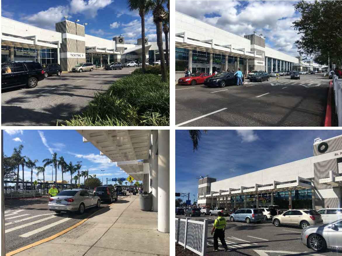
FIGURE 4.8-6: EXISTING CONDITIONS OF THE PRIMARY CURBFRONT DURING MIDDAY
