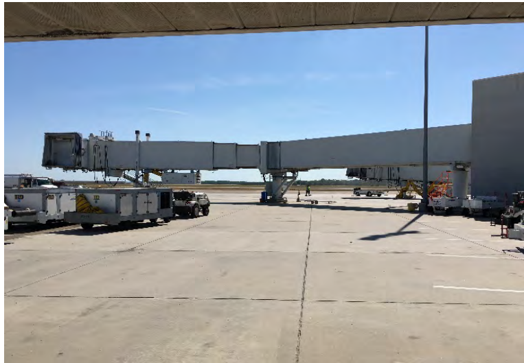
Gate 5 Passenger Boarding Bridge
